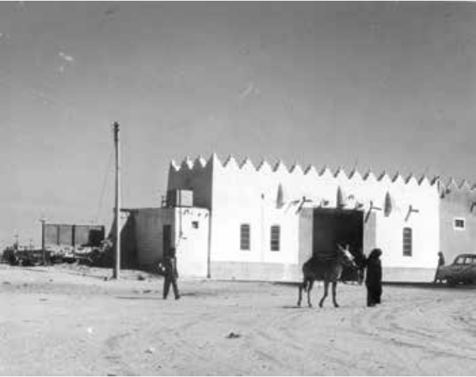
Kuwait Oil Company (KOC). A vernacular Kuwaiti house built with mud brick or rubble stone coated with thick mud plaster. The artistic touches were found on the main doors and windows, and the occasional geometric merlons along the roofline.
