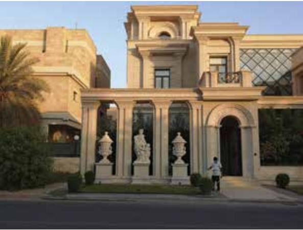
In contrast to the simple stone house on the left, this extravagant Kuwaiti home exhibits multiple dentil mouldings projected below the cornice level and hoodmolds around the doorway and smaller windows. Greco-Roman statues are placed on pedestals at the entrance and an ornamental iron railing on the balcony boasts the letter A. [Image courtesy of Ali AlYousefi (2020)].
